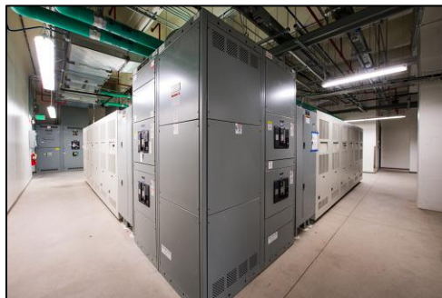
AC Grid Simulator (1MW, 600V)
