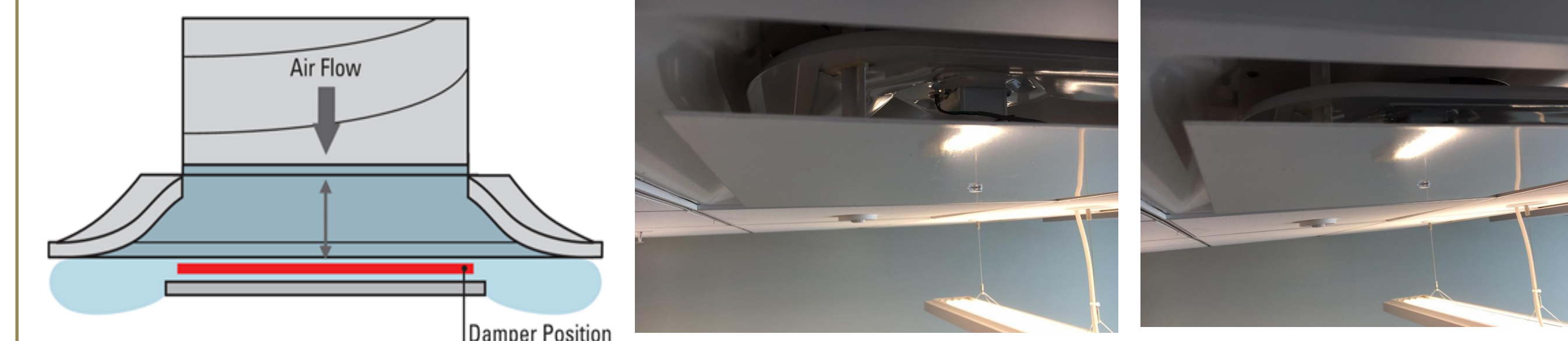
VAV diffuser with adjustable damper position
