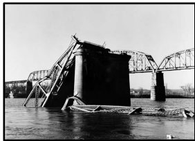
Silver Bridge Collapse (1967, West Virginia)
