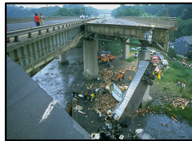
Mianus Bridge Collapse (1983, Connecticut)
