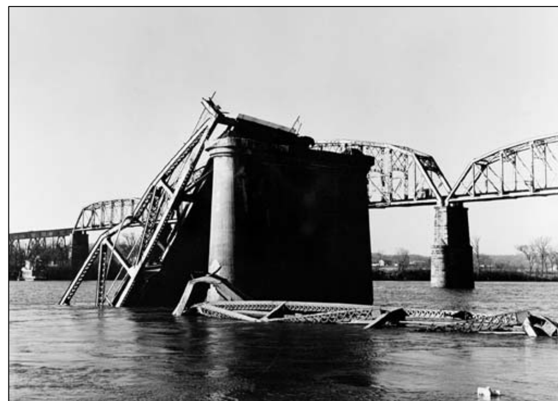
Silver Bridge Collapse (1967, West Virginia)
