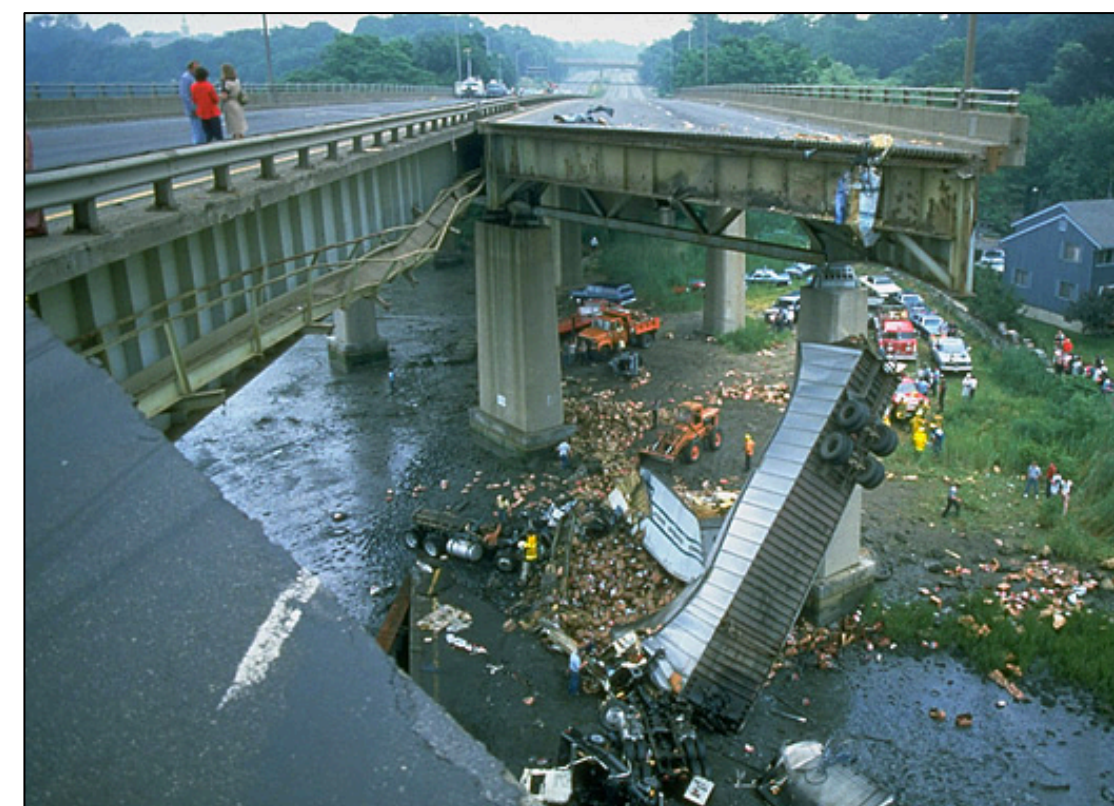
Mianus Bridge Collapse (1983, Connecticut)
