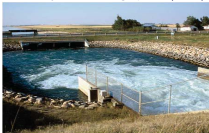
Tehama Colusa canal system (2007)
