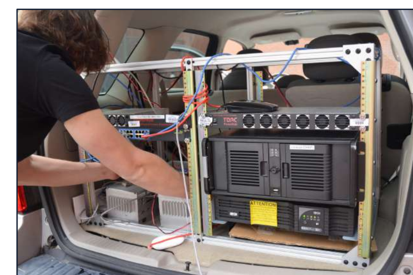
Sensors in the trunk of the CAT Vehicle that control the vehicle.
