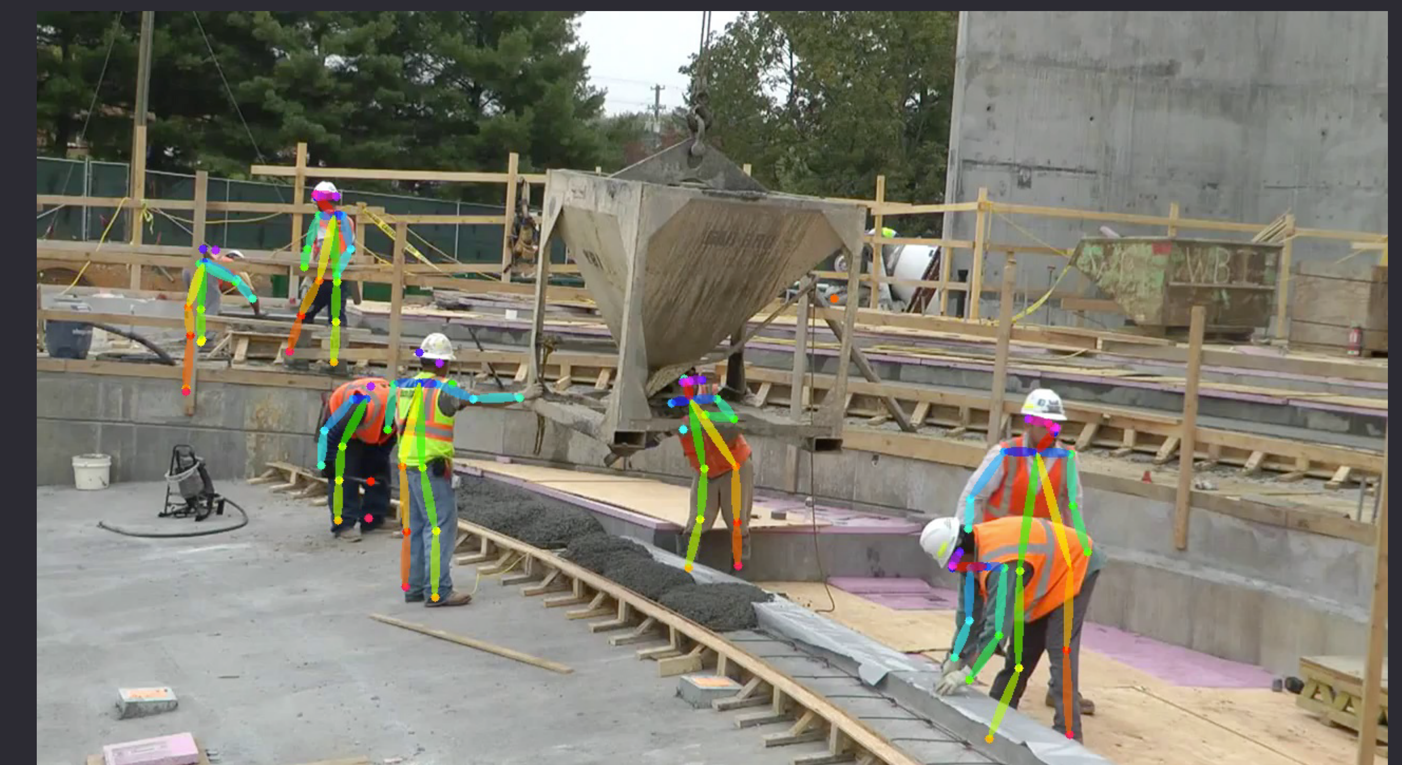
Tracking workers in real-time on a construction site and reporting both their pose and their proximity to other workers, equipment, and material in the scene for safety monitoring
