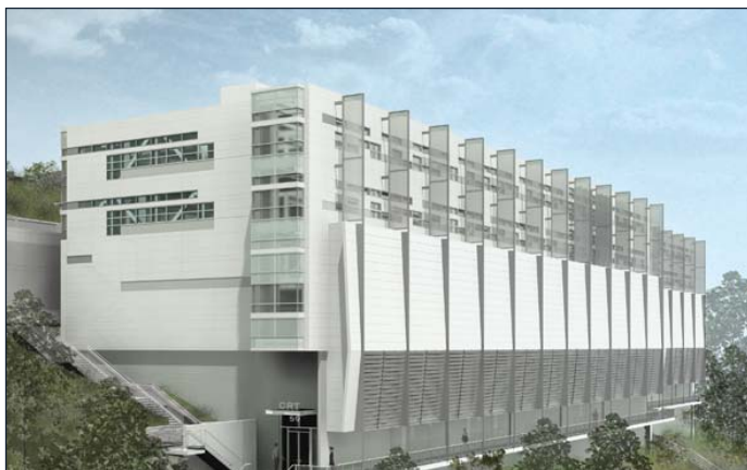
Computational Research and Theory Building will provide 12 MW power and cooling for future NERSC computing resources
