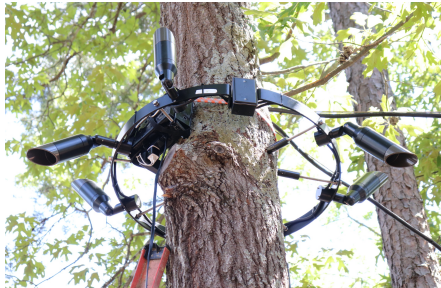
Fig. 1. Hardware system installed the Koka Booth Amphitheater in Cary, NC.
