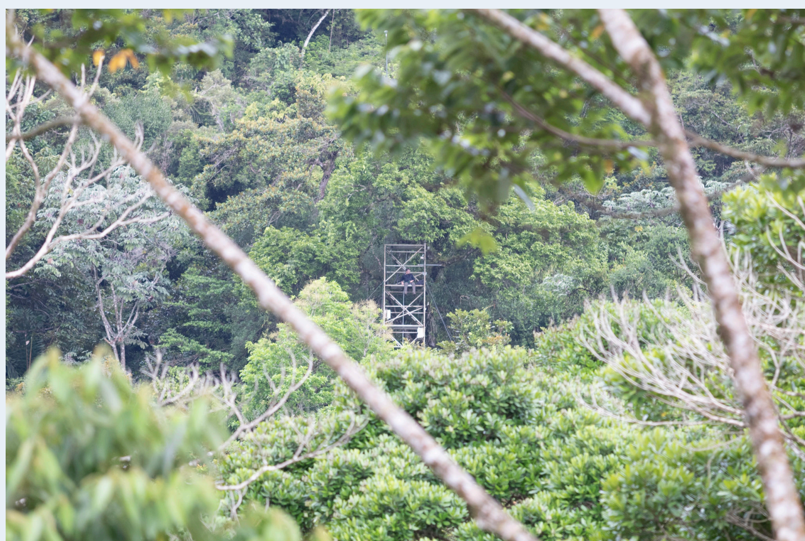
Example deployment terrain and tower.
