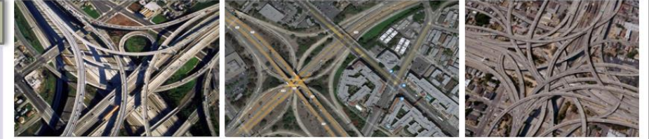
Complex and interconnected road networks
